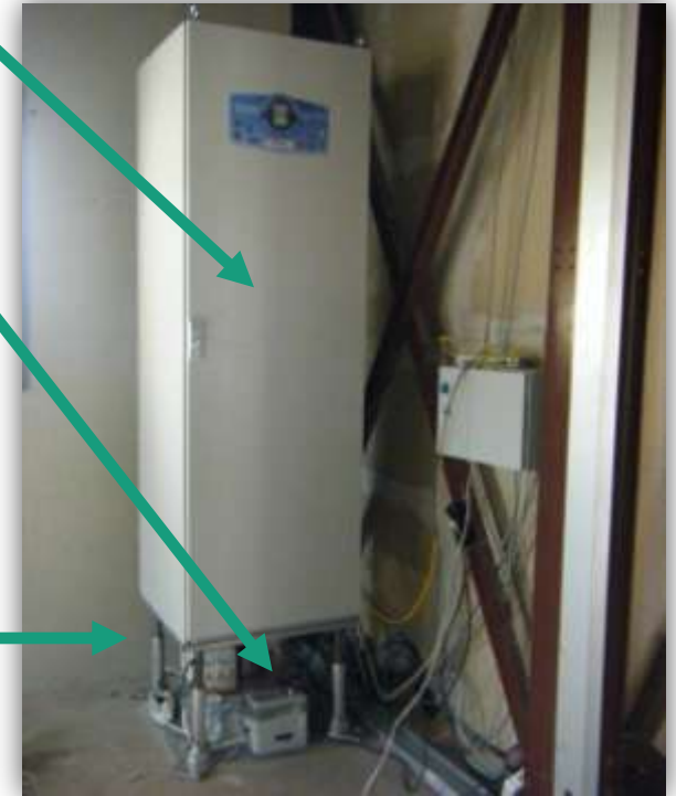
MR damping system installed
