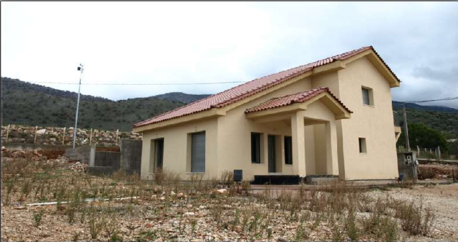
The Amfilochia demo house in mid-west Greece, constructed at the premises of Knauf Gypsopiia ABEE at Stanos-Amphilochia
