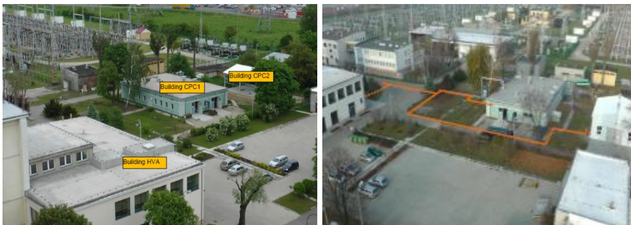
Figure 1. The demonstration industrial district setting in Warsaw, Poland. (left) location of each building in the district. (right) heat distribution network between the buildings.
